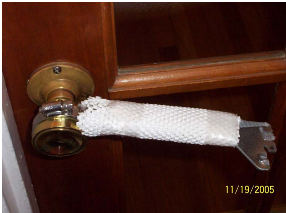
Figure 2.2: Protruding Part of Lever is Within Grasp of User
