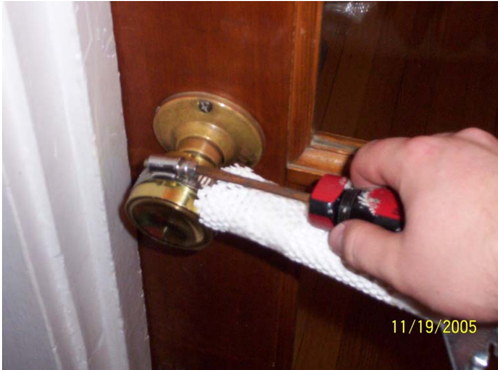
Figure 2.1: Securing Clamp to Door Handle with Screwdriver
